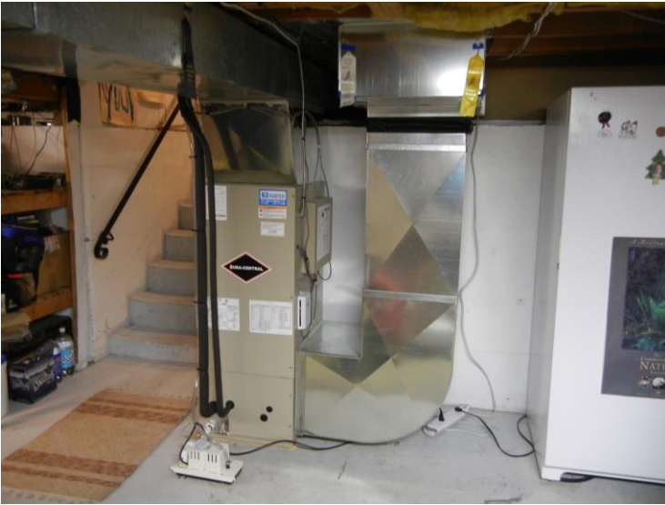
Internal Unit - Zuba Central ADP Air Handler 34,000 BTU
