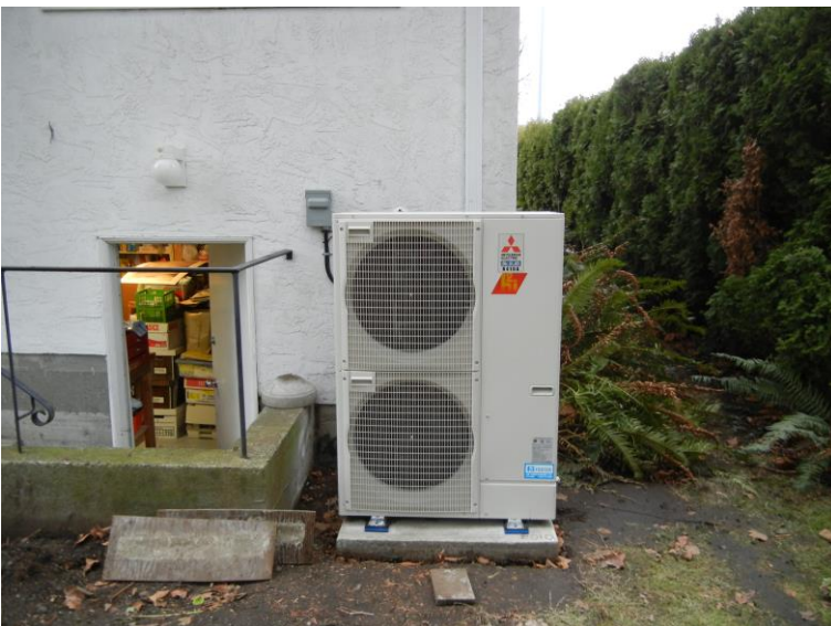
Exterior Zuba Central Unit - Mr Slim 34,000 BTU, HSPF
